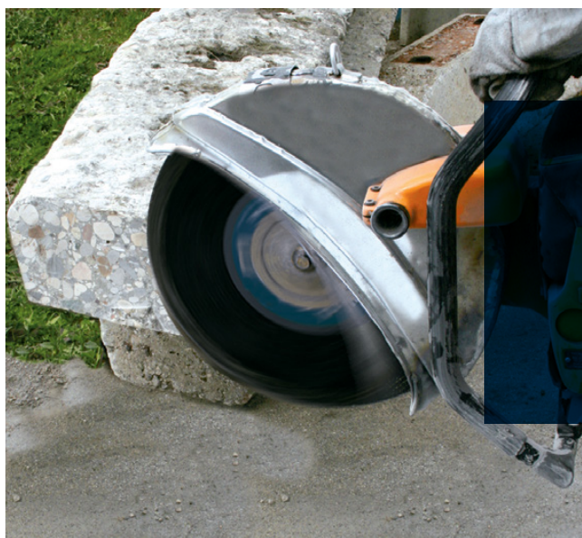
Metalynx PRO Stone wheel cutting a curb.
